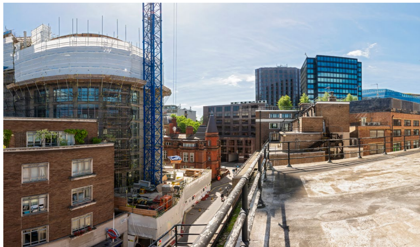
View from Palmer Street roof onto St James's Park Station
